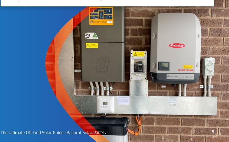
Larger residential systems may use either type, depending on the specific off-grid inverter and compatibility with solar inverters or solar charge controllers. The most modern inverters can accommodate both AC and DC coupling, offering a versatile and secure energy solution.
